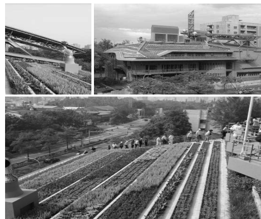
Figure 5 Sustainable extensive wild roof garden at the Magic School of Green Technology, National Cheng Kung University, Tainan, Taiwan.
