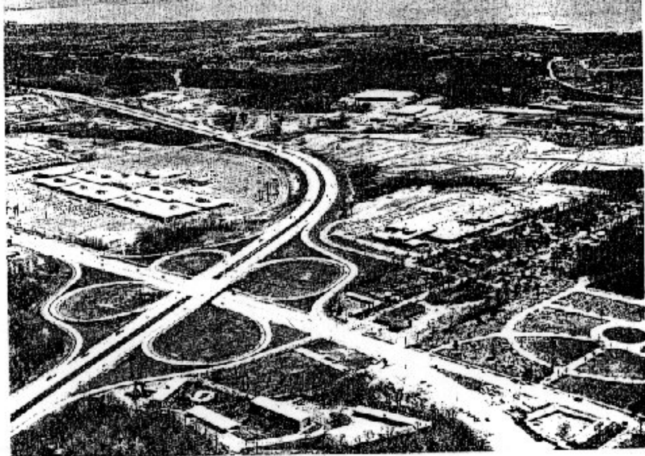
Plate 8.2 Millford Center, Milford, Connecticut, USA. Located in the fast growing suburban zone outside New York City, this is a good example of the suburban, edge-of-town, new shopping centres that have developed on a large scale for car-based shoppers in the United States since the Second World War.
