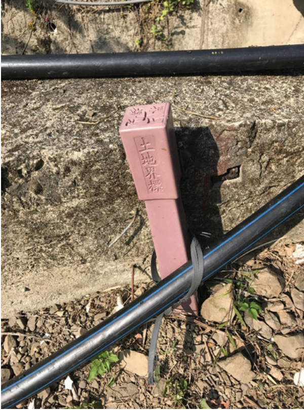
Figure 5: Land boundary marker and a pipe attached on it in the edge of a field.
