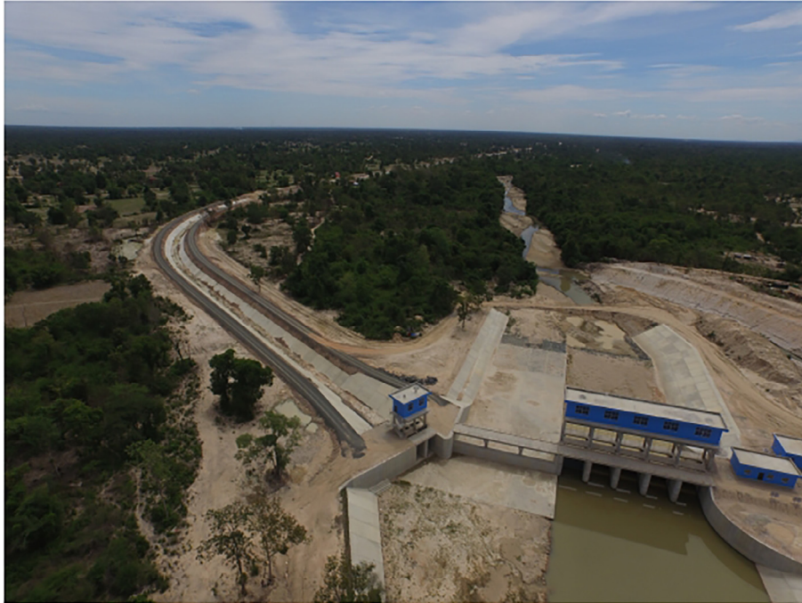
Fig. 4. Sinohydro dam under construction. Drone photo: V. Rong, June 5 2016.
