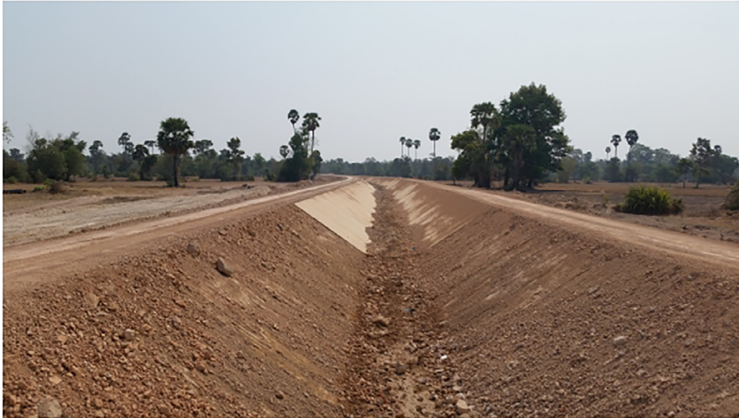
Fig. 3. Sinohydro canal under construction. Photo: C. Work, June 5 2016.
