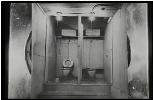
112. Photograph of Two Toilets (22:45-24:03)
