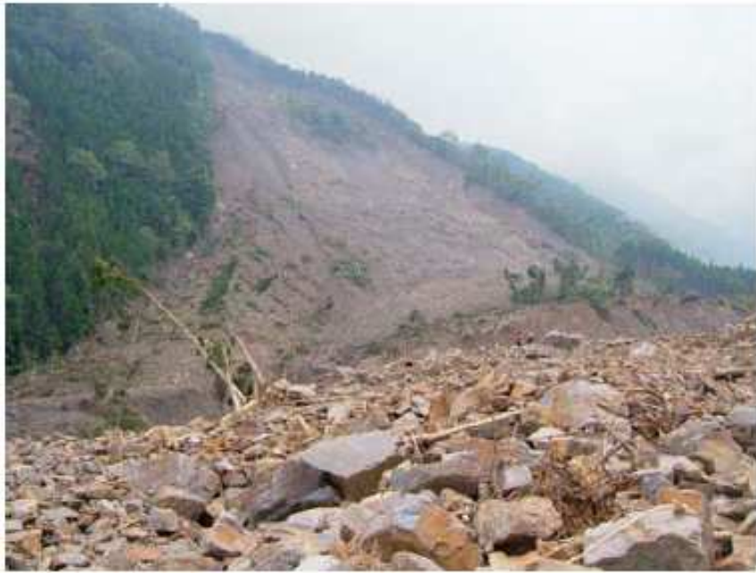
Figure 4-3. Mudslides in Taoshan Village after Typhoon Aere Source: Soil and Water Conservation Bureau Council of Agriculture
